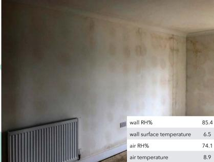
Black mould and straining is clearly visible and penetrating through the paint coat.
