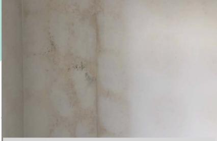
Even after use of stain blocker and repainting the wall several times the mould and staining is still clearly visible.
