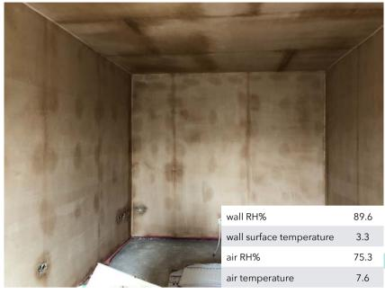
Skim-coat applied to dot and dabbed plasterboard. Substrate - block work The substrate is not suitable for application of any typical emulsion paint.
